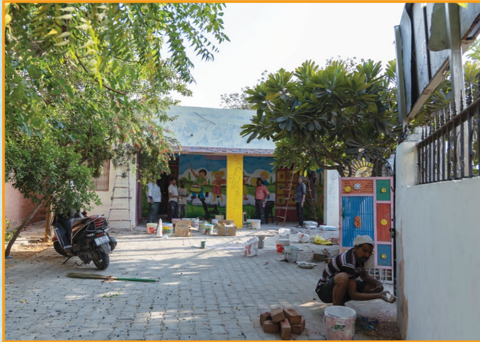
The ongoing restoration work at the Khanpur Khurd Anganwadi is laying the foundation for a brighter tomorrow for the community's youngest members.
