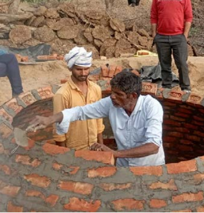
Construction of a biogas plant in Bass Village, Rewari, Haryana.
