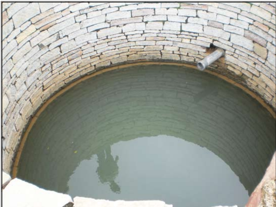
Figure 9: Abandoned and failed wells are successfully retrofitted as rainwater recharge and storage units- highly useful in water scarce regions
