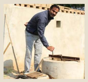
After feeding the plant with dung, it took a few days to produce the gas. In the beginning, the plant started producing ammonia gas, which is not inflammable. A biogas plant should produce methane gas. He opened the tank, to release the gas and empty the plant. After that, he added a sack full of jaggery to the tank. Jaggery is inflammable and when mixed with cow dung, it helps in producing gas. In a few days, the plant started producing methane gas and functioning smoothly.
