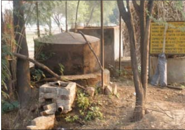
P19: KVIC model biogas unit
