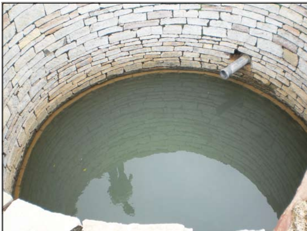
Figure 9: Abandoned and failed wells are successfully retrofitted as rainwater recharge and storage units- highly useful in water scarce regions
