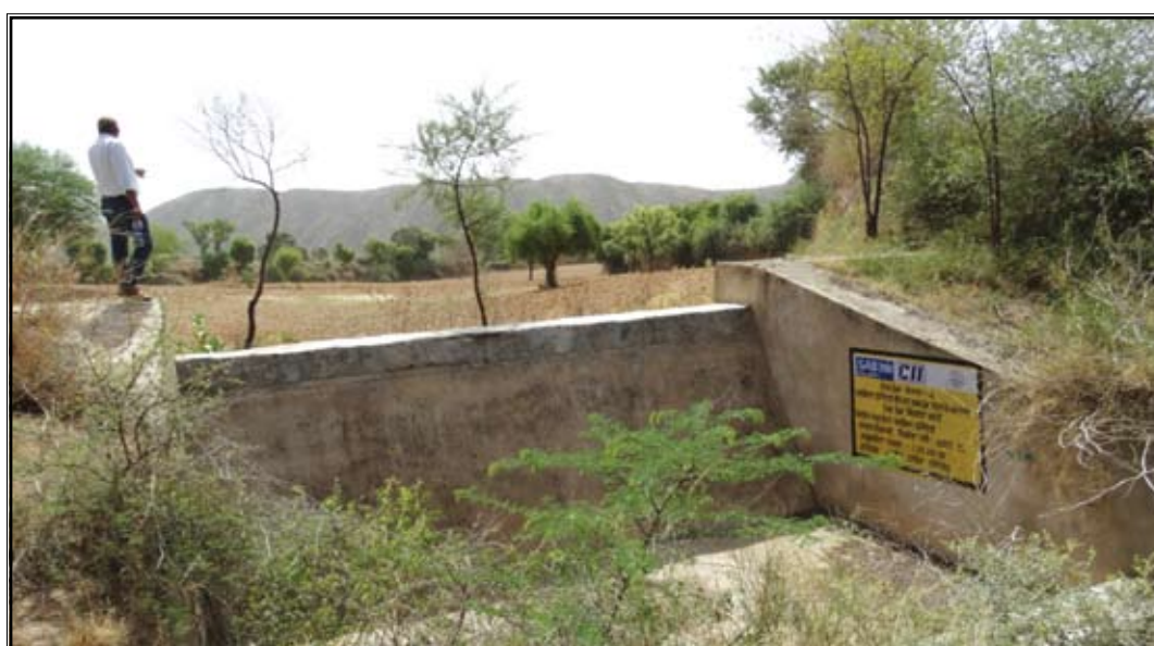
Figure 5: Levelling of undulating gullies and construction of check dam has enhanced both the cropped area and the crop productivity in Silarpur, Neemrana block
