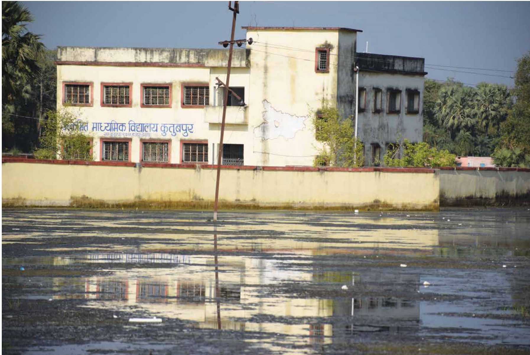
The flooded precincts and surroundings of a part of the Government Middle School in Qutubpur, Bihar. Three light green fruit trees planted within the boundary of the school can be seen in the picture. With the area flooded for months, the survival of these trees remains precarious.
